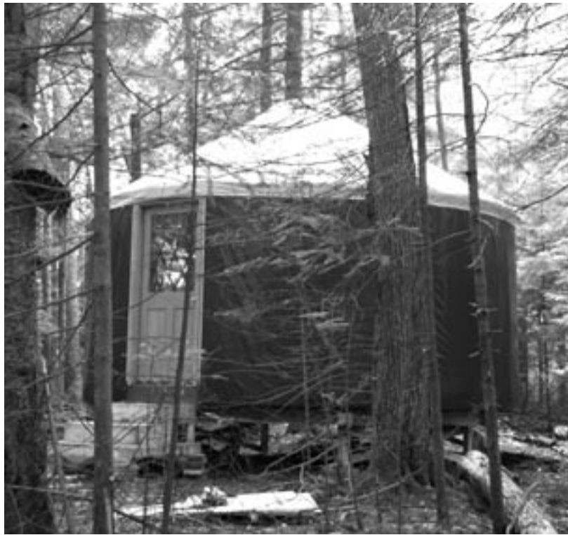
The first of several to be erected, Camp's new yurt is green with a cream roof and beautiful insulated wood door.
